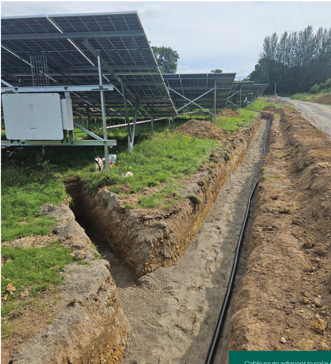
Cable route adjacent to solar panel arrays. Credit: Statkraft
