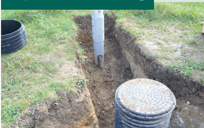
CCTV post installation. Credit: Pre-Construct Archaeology
